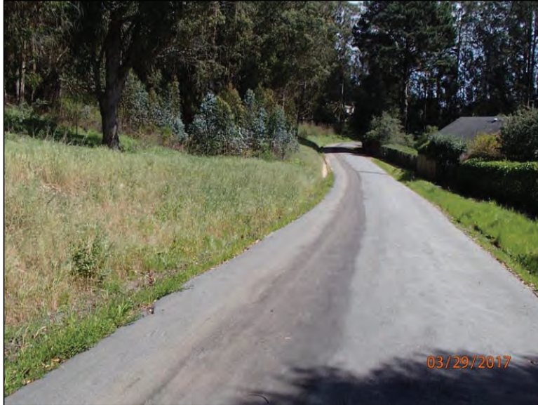
Photo 37 (Urban Drainage Interface – AOC 3): View of the urban drainage interface located on Moro Ave, (AOC 3, Map 2). Flow is conveyed down the inboard ditch for ~325' to a ditch relief culvert at the intersection of Santiago Ave. and Moro Ave. The crowned road surface keeps the majority of the stream flow on the inboard edge of the road.
