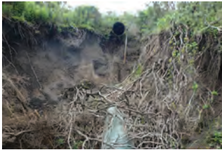
Erosion repair example
