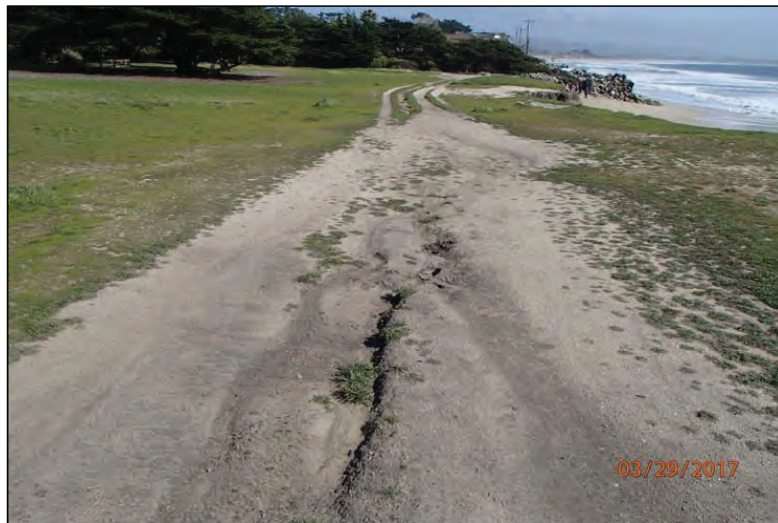
Photo 32 (Coastal Bluff Trail): View of road surface erosion along the coastal trail due to concentrating runoff. Note the exposed beach protection rock armor at the edge of the park boundary in the distance.
