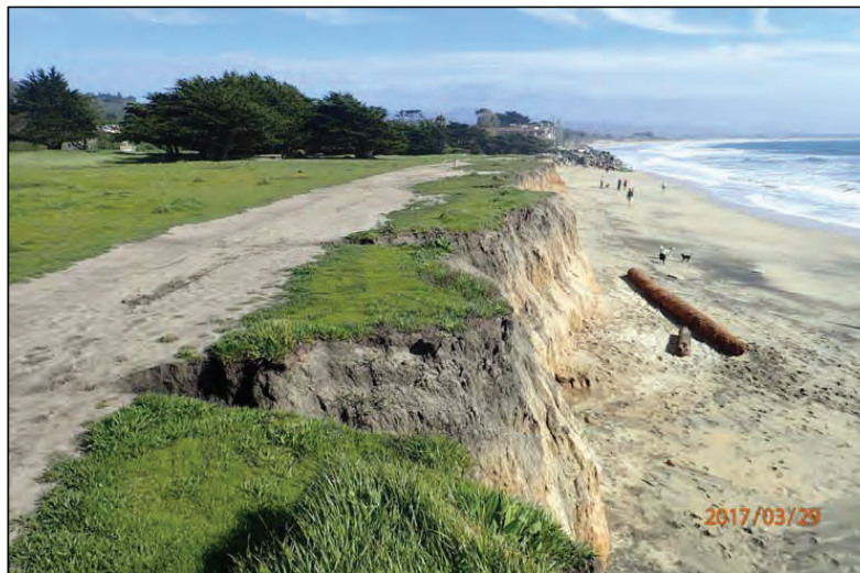
Photo 30 (Coastal Bluff Trail): View of bluff retreat looking south along unpaved coastal trail. The gullies located along the wave cut bluffs are exacerbated by concentrated runoff from the trail and upslope marine terrace meadows.
