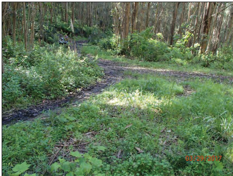
Photo 28 (Site #38): View of the right road approaches to a fill on crossing on a Class III stream on the South Ridge Trail.
