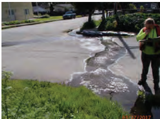
Run-off into residential areas
