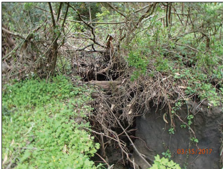
Photo 10 (Site #2): View of an active 5.5ft tall headcut at the downstream extent of the inundated pond at stream crossing Site #2 on the Meadow trail shown in the previous photo.
