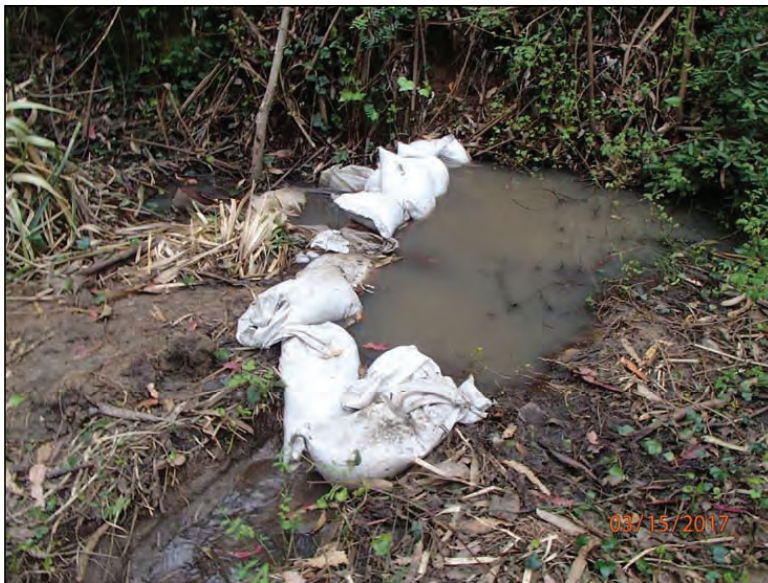
Photo 6 (Site #4): View of temporary dysfunctional sandbag spillway at the southwest corner of the on-stream pond Site #4.
