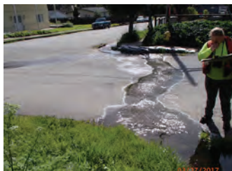
Run-off into residential areas
