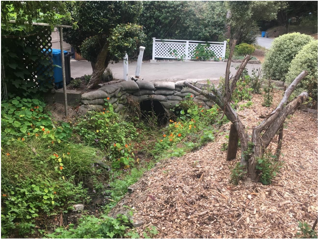
Photo B-2. View of Dean Creek looking west with culvert under driveway. Photo date: 7/20/2018.
