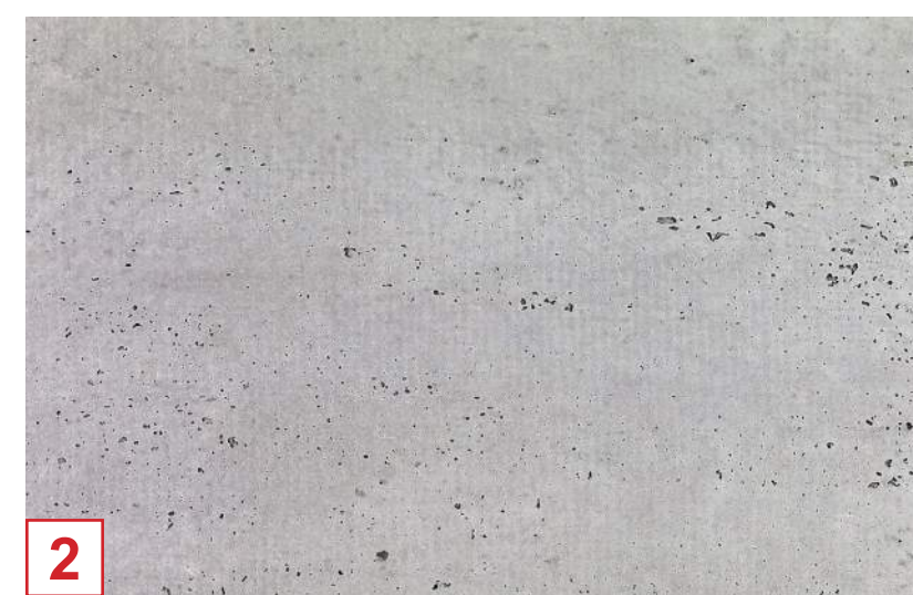
2 EXTERIOR ENVELOPE & WALLS CONCRETE
