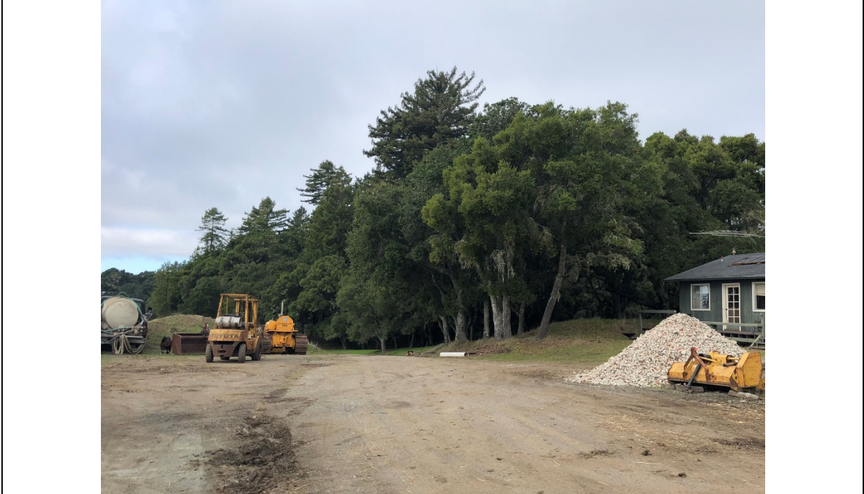
Photo 2. Existing development area including house, barn, staging area, and access road.
