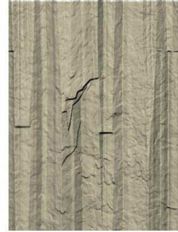
CONCRETE WALL FINISH: BASALT LINER STAINED
