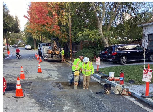
Image 1 - Construction Activities in the ROW
