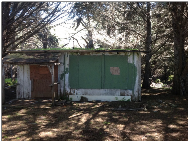
Photo 8: Unused cabin near the landslide area
